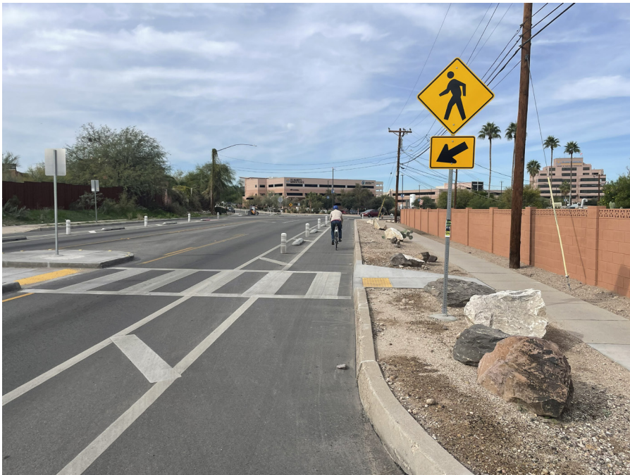
A separated bike lane in Tucson, Arizona provides dedicated space and vertical separation by using delineator posts and pre-cast concrete curb.
