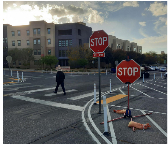
Signage, flexible delineator posts, traffic paint, and detectable warning surfaces can enhance crossings.
