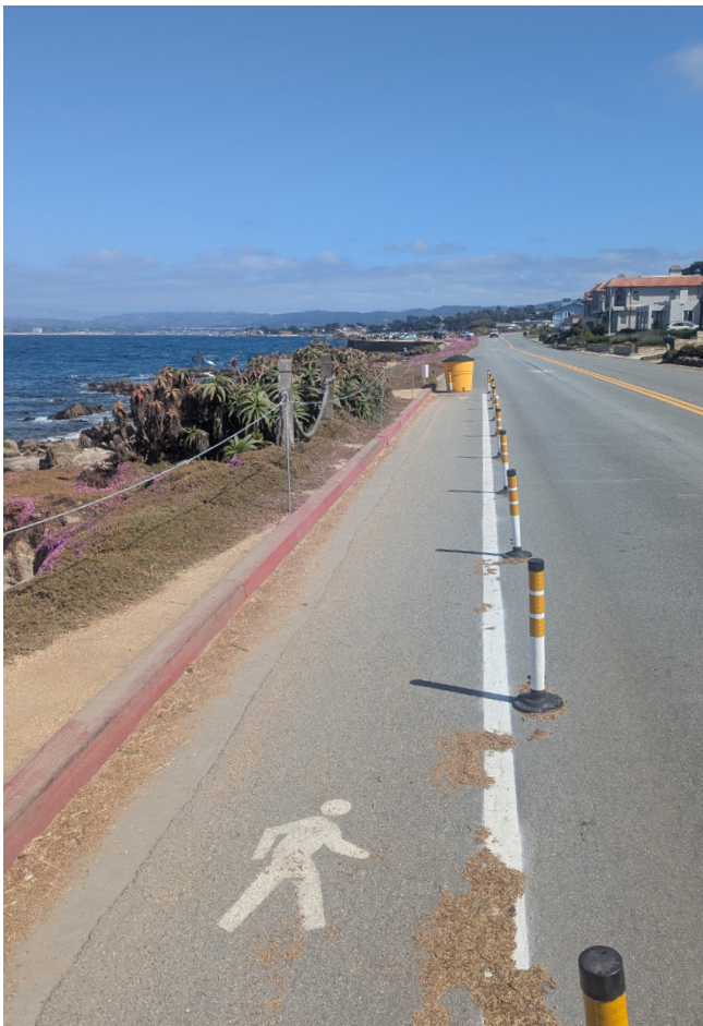
A pedestrian lane fills a short gap in an off-street trail through constrained conditions in Pacific Grove, California.
