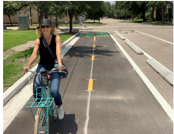
Pre-cast concrete curbs and traffic paint can define the edge of separated bike lanes and other facilities.
