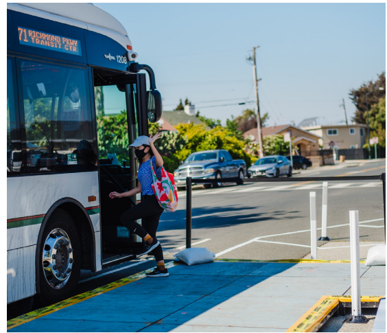
Modular bus stop platforms can create accessible transit stops within the roadway pavement section.
