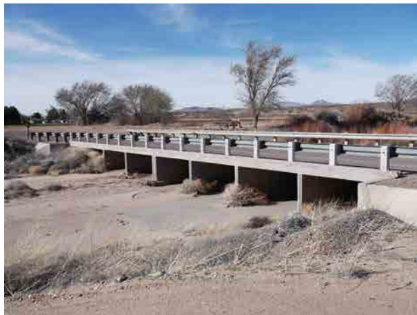
Box culvert at the Placitas Arroyo and Canal Road crossing
