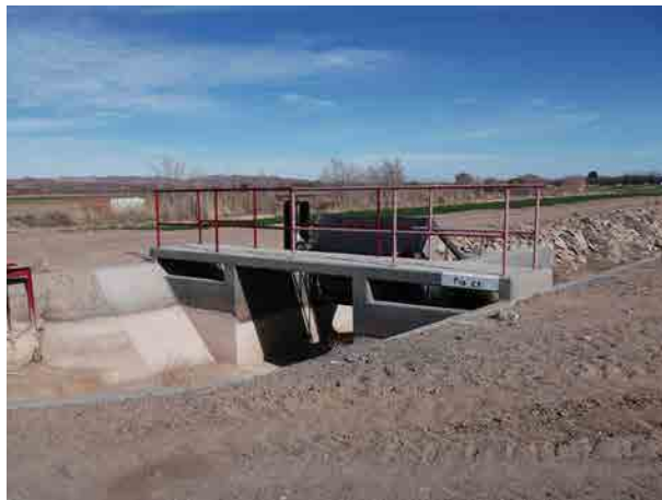
Elephant Butte Irrigation District Radial Sluice Gate at the Placitas Arroyo
