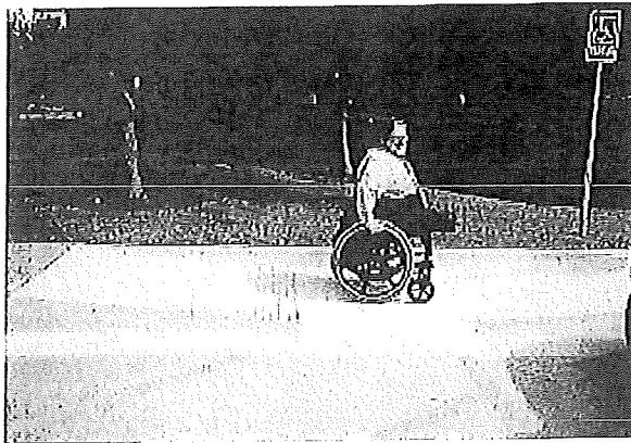
Figure 7-37. Parallel curb ramps work well on narrow sidewalks but require users continuing on the pathway to negotiate two ramp grades.
